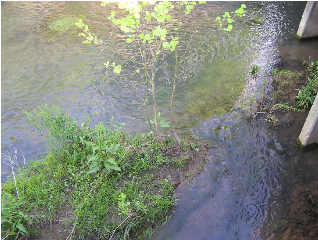
Photo 7: STA 138+00 LT, view of STR-3 facing west.
