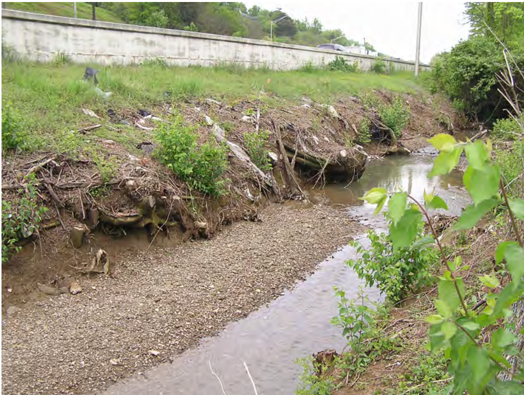
Photo 2. STA 120+00 LT, view of STR-1 facing southwest.
