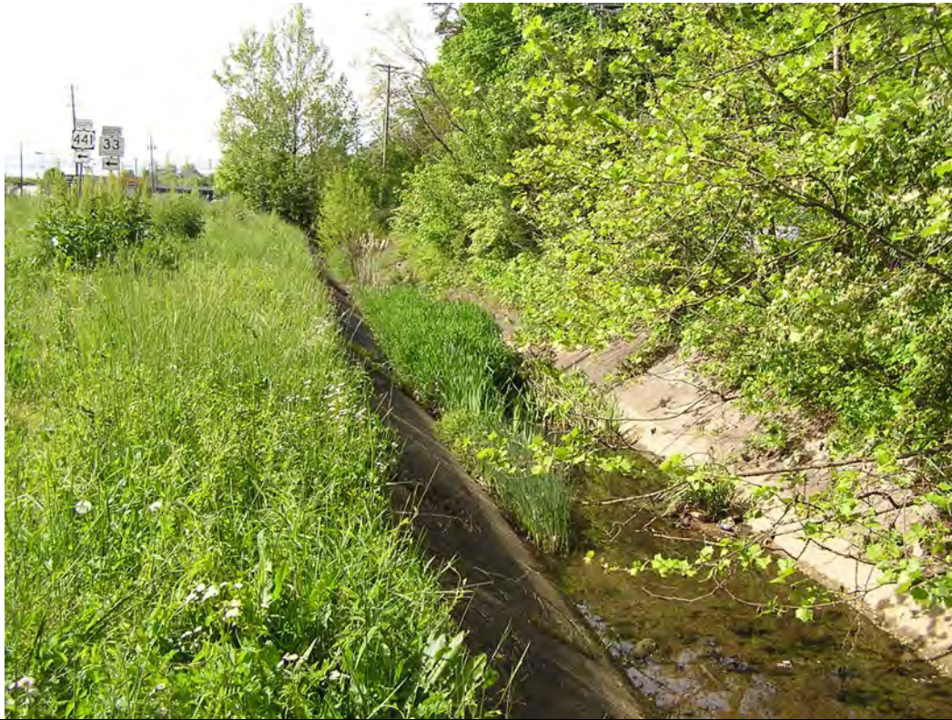
Photo 9: STA 60+00 LT, (Tazewell pike), View of STR-4 facing south.
