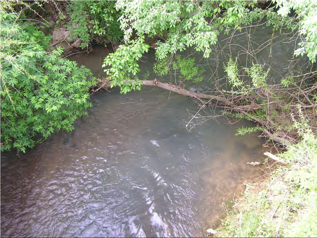
Photo 11: STA 152+50 RT, View of STR-5 facing west.
