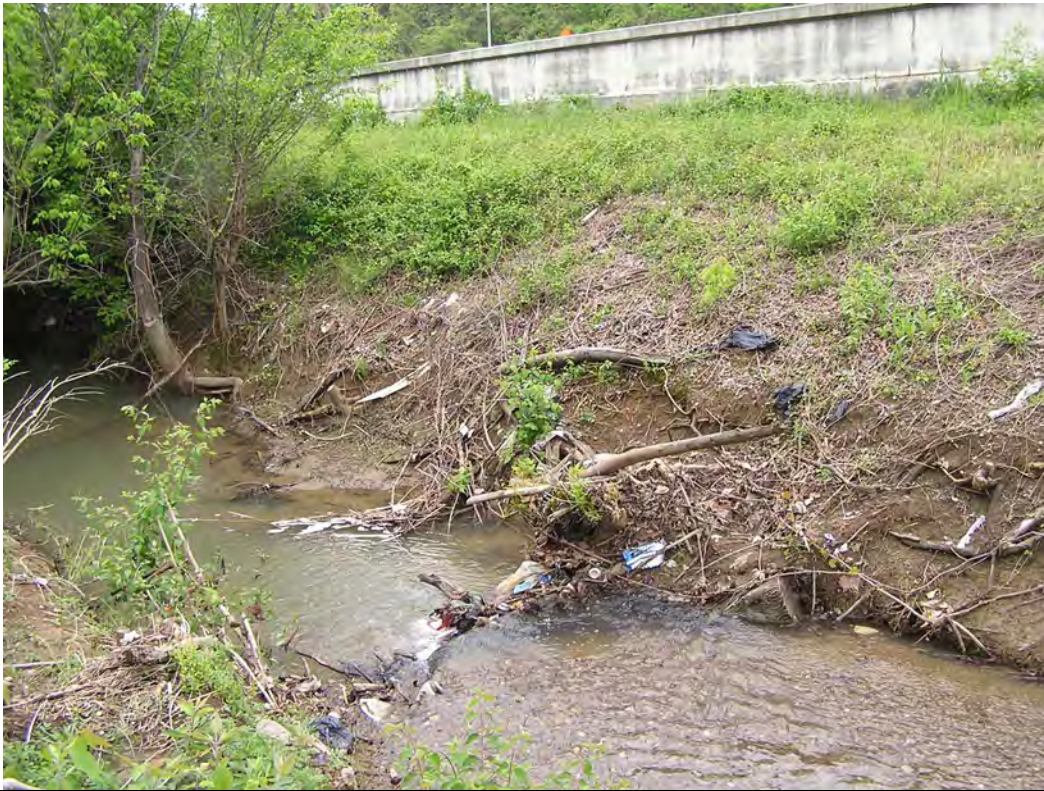
Photo 1: STA 120+00 LT, view of STR-1 facing southeast.
