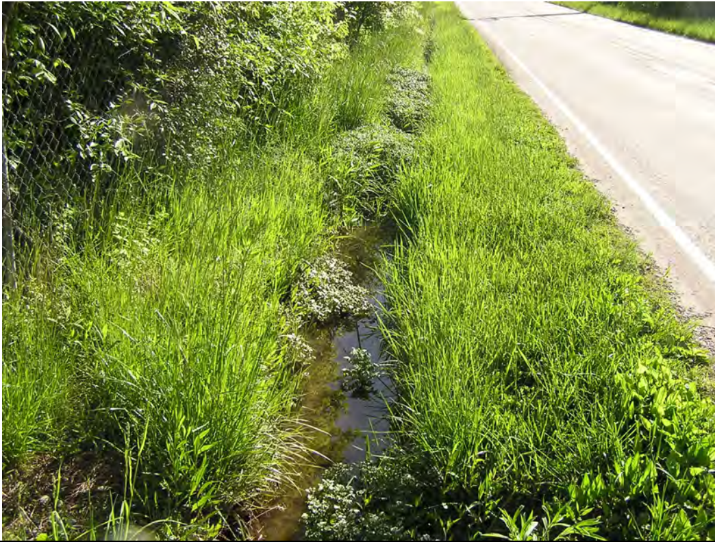
Photo 3: STA 115+00 LT, view of STR-2 facing southeast.
