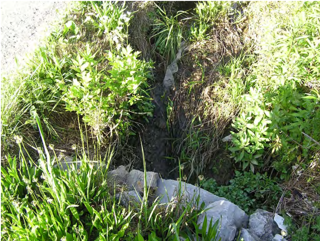
Photo 4: STA 113+00 LT, view of STR-2 facing southeast.
