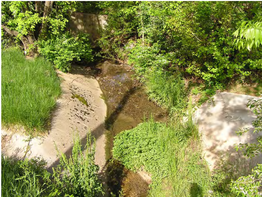
Photo 10: STA 522+00 RT, (Old Broadway), view of STR-4 facing east.
